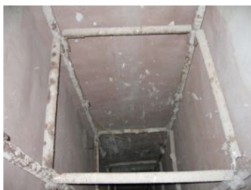
The Lift Shaft
